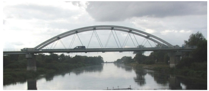
Figure 3. The road bridge over Noteć river in Santok (Poland) - (Nadolny G. 2005)
