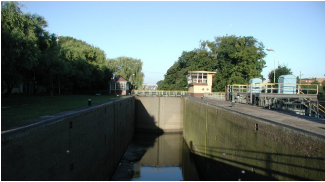
Figure 1. The lock in Czyżykówko on Wisła – Odra waterway
