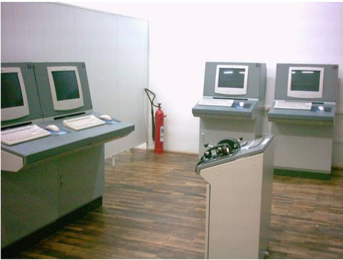
Figure 3. Local Control Room with 4 Local Operating Stations (LOS)
