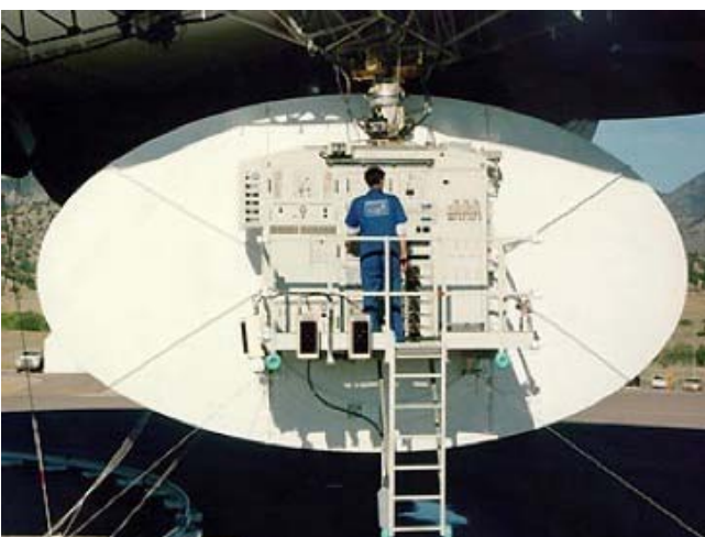
Figure 5. Rotational radar antenna under maintenance
