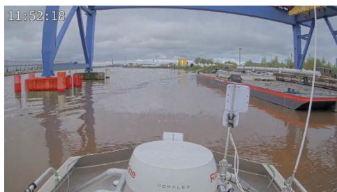
Figure 1. Crane in the Jarßum Harbor in Emden, as seen from the research vessel. The crane foundation on the left side is marked in red.
