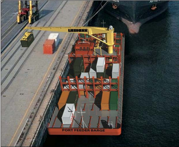
Figure 4. Port Feeder Barge is working independently from quayside equipment at a deep sea terminal requiring only a small gap between two deep sea vessels
