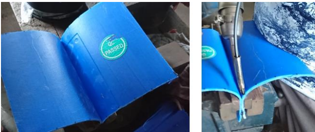
Figure 4. Joining two layers of HDPE sheet by HDPE welding
