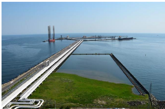
Figure 4. Actual construction of Oil Terminal in Northern Port of Gdansk [1]
