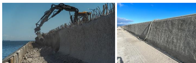
Figure 8. Case study 2, Left: Repair works on the seaward wall of the Northern Island Breakwater. Right: View of the repaired parapet of the Northern Island Breakwater from the inner side showing shotcrete coating on the parapet and surface sealing with spray applied polymer-cement coatings, source: own
