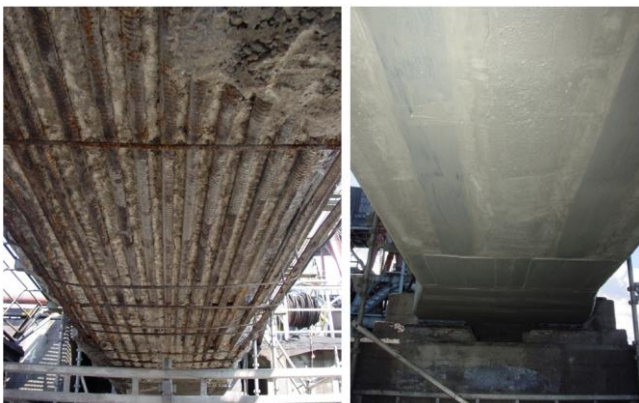
Figure 20. Case study 6, Left: after removal of loose or poorly bonded concrete fragments; all reinforcement bars of the bottom layer are visible. Right: the same element during repair - application and anchoring of carbon fiber tapes, source: own
