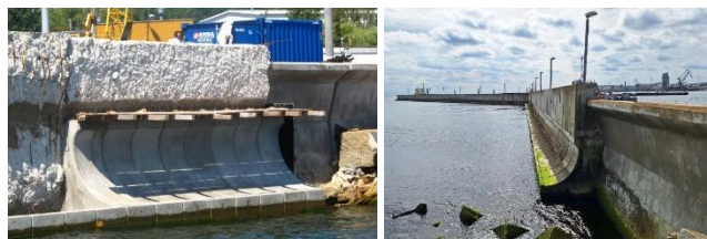
As a result, a full-scale rehabilitation of the seaward face of the head section was undertaken in 2012. The repair involved breaking down the damaged concrete parapet between +2.20 m and +0.70 m to a depth of 30 cm, followed by the installation of prefabricated reinforced concrete facing panels and the construction of a new parapet within this protective shell. The new parapet was cast from C30/37 concrete and reinforced with BS500S ribbed steel bars ( \phi 12 mm and \phi 16 mm), with a specified concrete cover of 70 mm. The seaward wall was formed using prefabricated panels, while the port-facing side was coated with shotcrete made of C30/37 concrete, (Fig. 2, Fig. 3).
