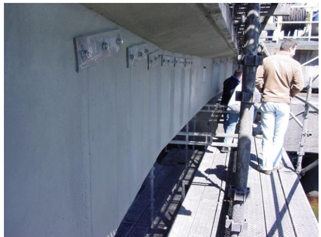
Figure 23. Case study 6, Application and anchoring of carbon fiber mats, source: own
