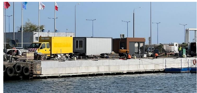
Figure 17. Case study 5, View of the mooring and fender line after reconstruction, with the GRC prefabricated element visible on the quay wall, source: own
