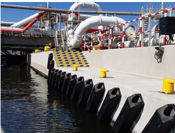
Figure 11. Case study 3, View of the modernized structure after reconstruction, source: own
