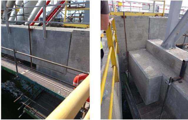
Figure 14. Case study 4, Condition of the platform after renovation, source: own
