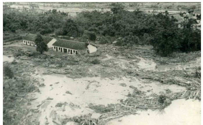
Figure 5. Destruction in the dock area and Packing House of English Farm after the debris flow of March 1967.
