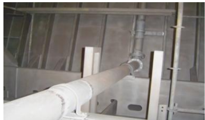
Figure 5. Sand blasting of the inner surface [16]
