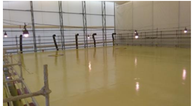
Figure 17. Surface after paint application
