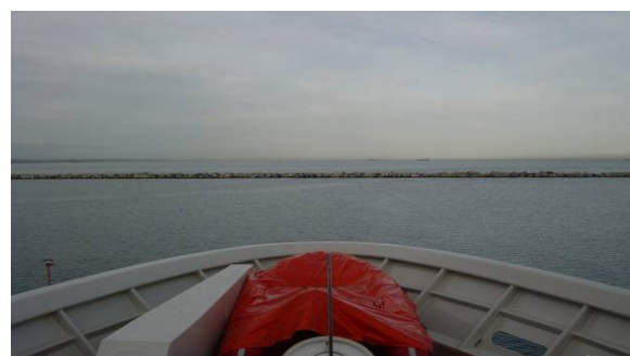
Figure 7. Breakwater in front
