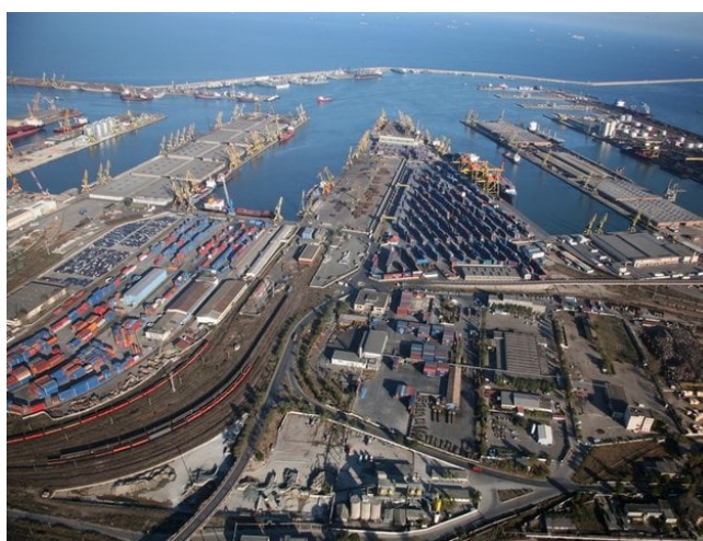
Figure 3. Constanța South Container Terminal (aerial view) [4]
